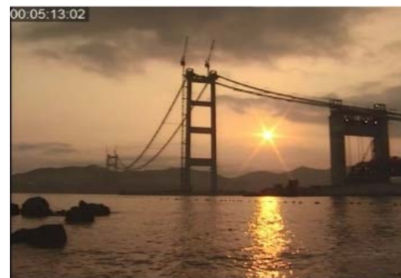
Tsing Ma Bridge under construction in the sunset (Reference no.: HKRS 2693-1-165)
