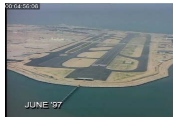
The airport at the last stage before completion (Reference no.: HKRS 2693-1-393)
