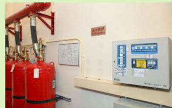
FM200 Fire Suppression System in all repositories
