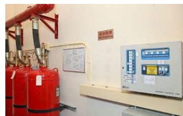
FM 200 Fire Suppression System in all repositories
