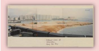
Phase I of the reclamation work of Hung Hom Bay commenced in 1986. After completion of the work. an area of approximately 20.5hectares of foreshores and sea-bed at Hung Hom Bay created for were the purpose of expanding the
