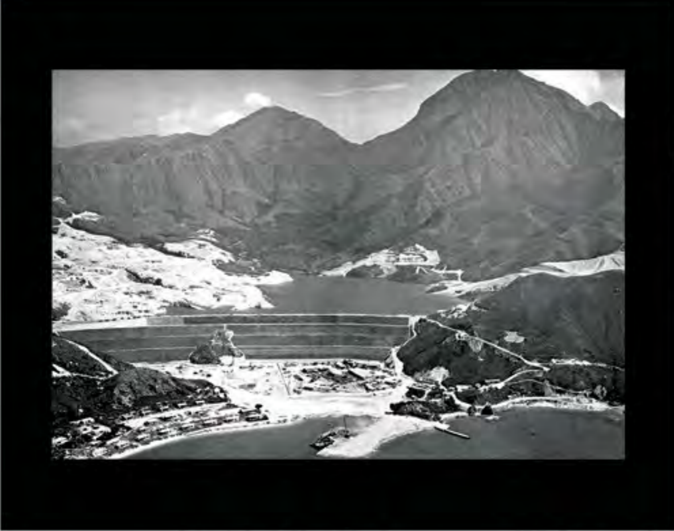
1967年的石壁水塘。水塘的建造費為2.2億元，儲水量為53.9億加侖。 Shek Pik Reservoir (1967). The construction cost of the reservoir was $220 million and it's storage volume was 5,390 million gallons.
