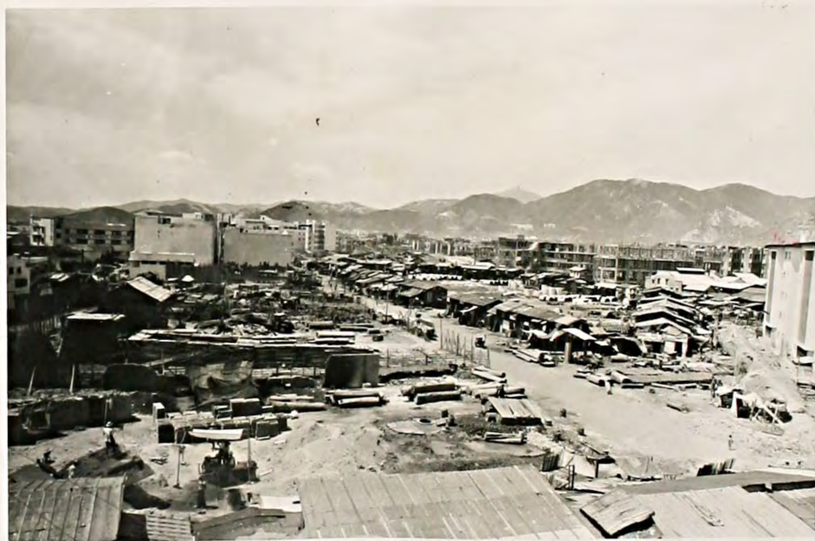
310/2 Full view of the surveyed area supplementary to 310/1.
