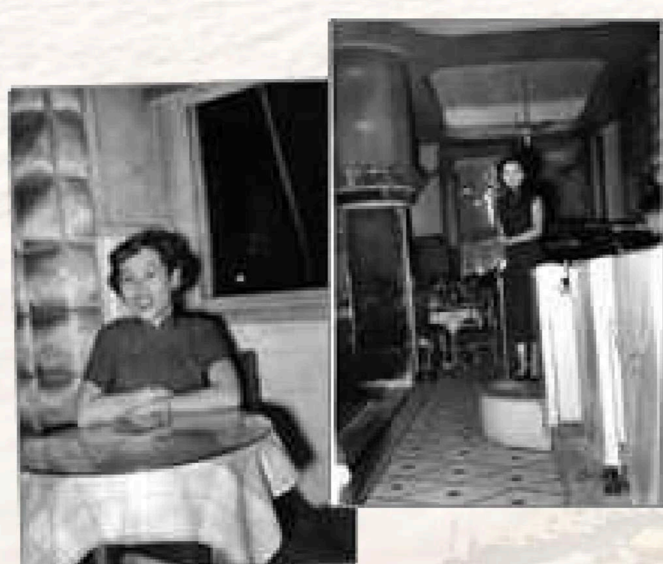
Interior of Hennessy Ballroom (1950s)
