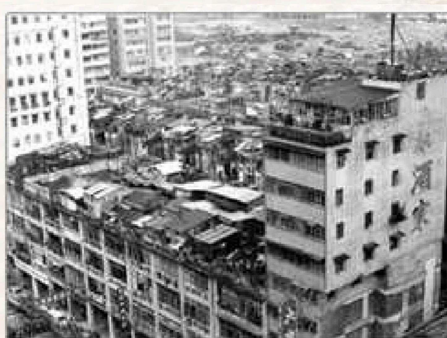
Tenements and roof-top huts along Lockhart Road. Wan Chai Reclamation (top) is almost completed (1970)
