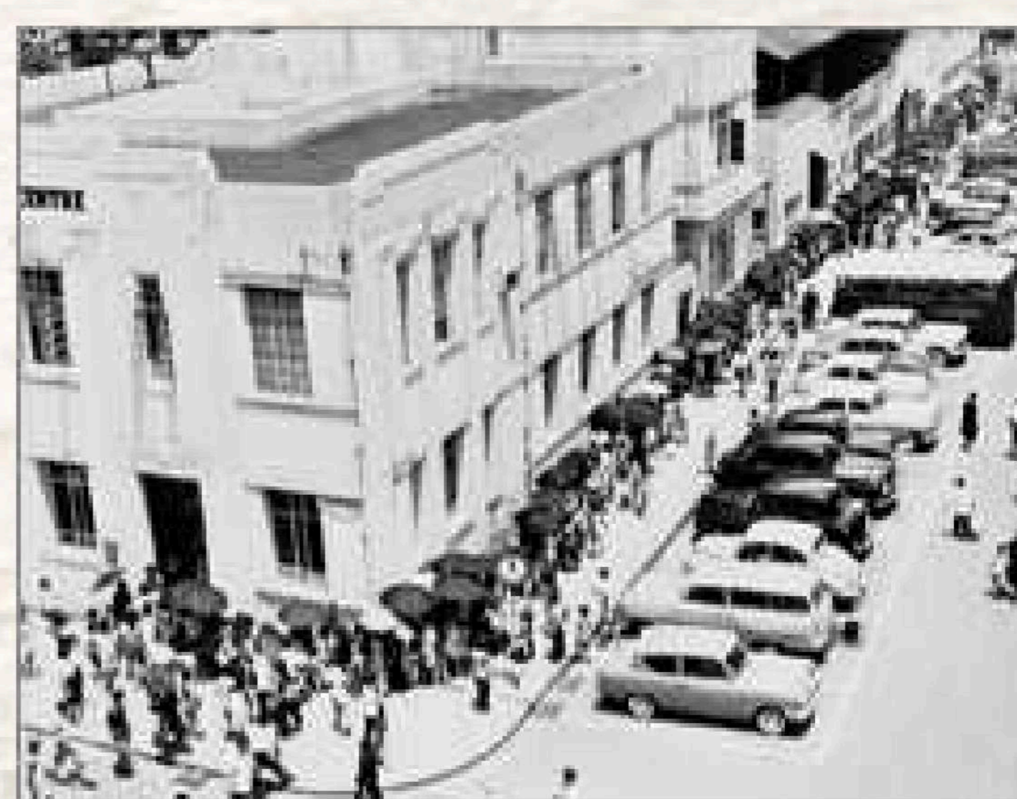
Violet Peel Clinic at the junction of Johnston Road and O'Brien Road (1960s)
