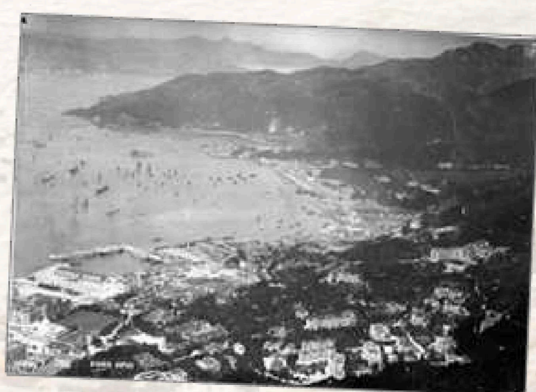
View of the newly-completed naval dockyard, Wan Chai and Causeway Bay (c.1910)
