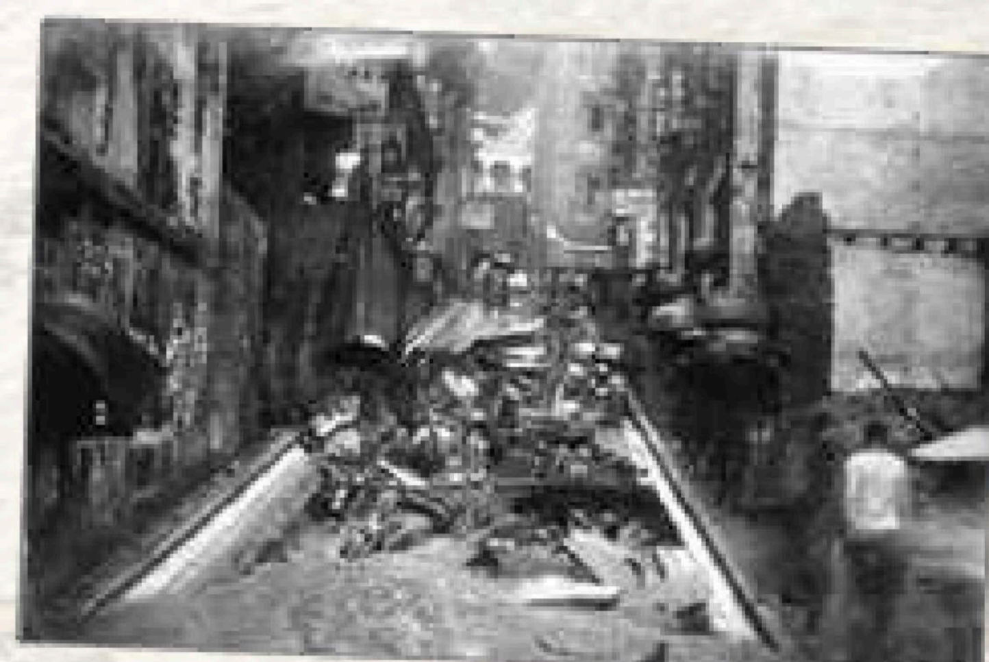
St. Francis Street after a heavy rainstorm (1926)
